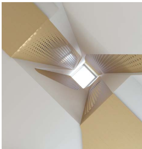
View of the Inner Courtyard and skylight
