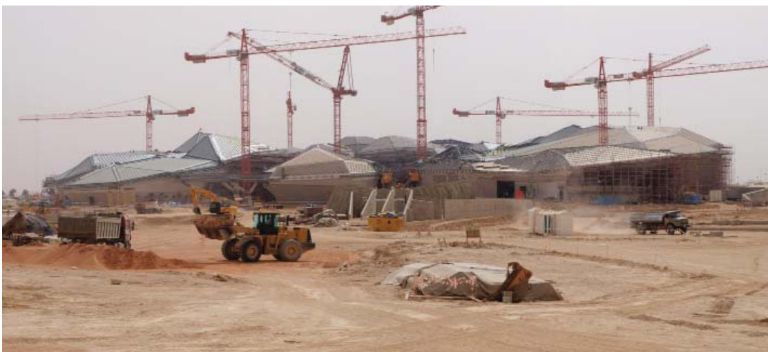
KAPSARC: construction site April 2013
